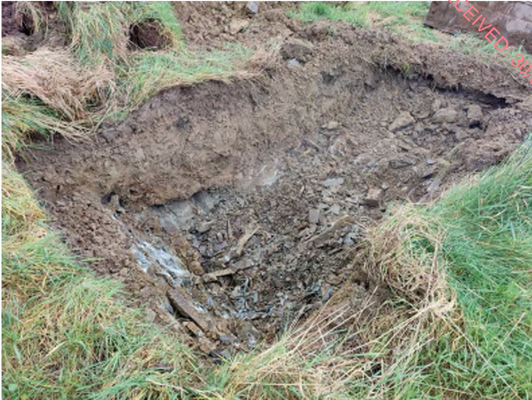
REXTP02 – 2 of 6 Bucket excavation to 0.80m
