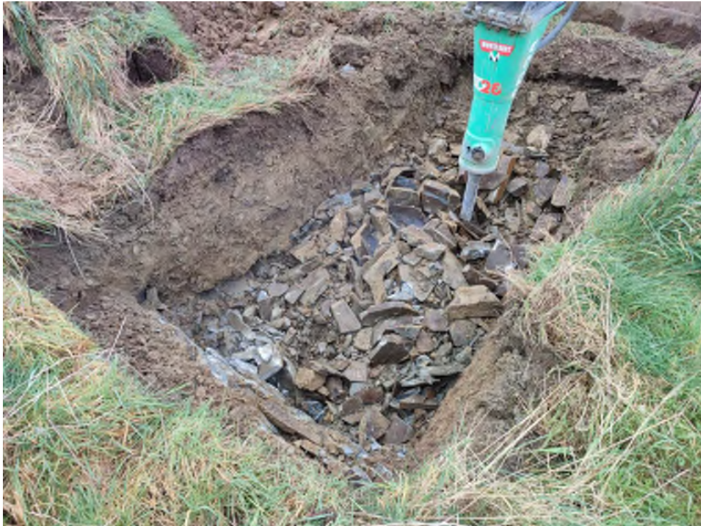
Figure 9 – Hydraulic breaking in REXTP02
